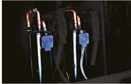
Multiple large-capacity all inverter compressors (more than 14 HP).
