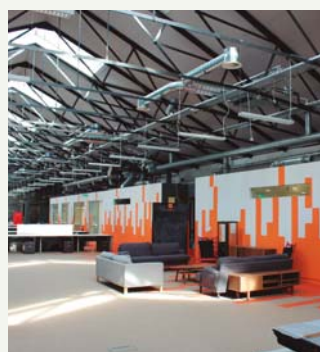
Zalando's solution for its warehouse office conversion at Grand Canal Quay, Dublin. ECOi
