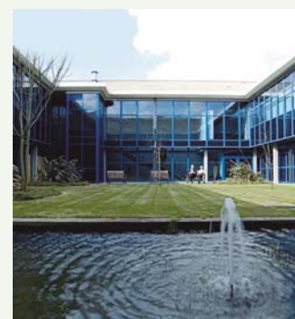
NHS Canford house clinic, Bournemouth, UK. VRF
