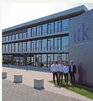
ITK Engineering GmbH. An innovative office building located in Germany. ECOi - PACi
