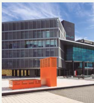
Andalucia Technology Park. Offices of high energetic efficiency. Spain. ECOi
